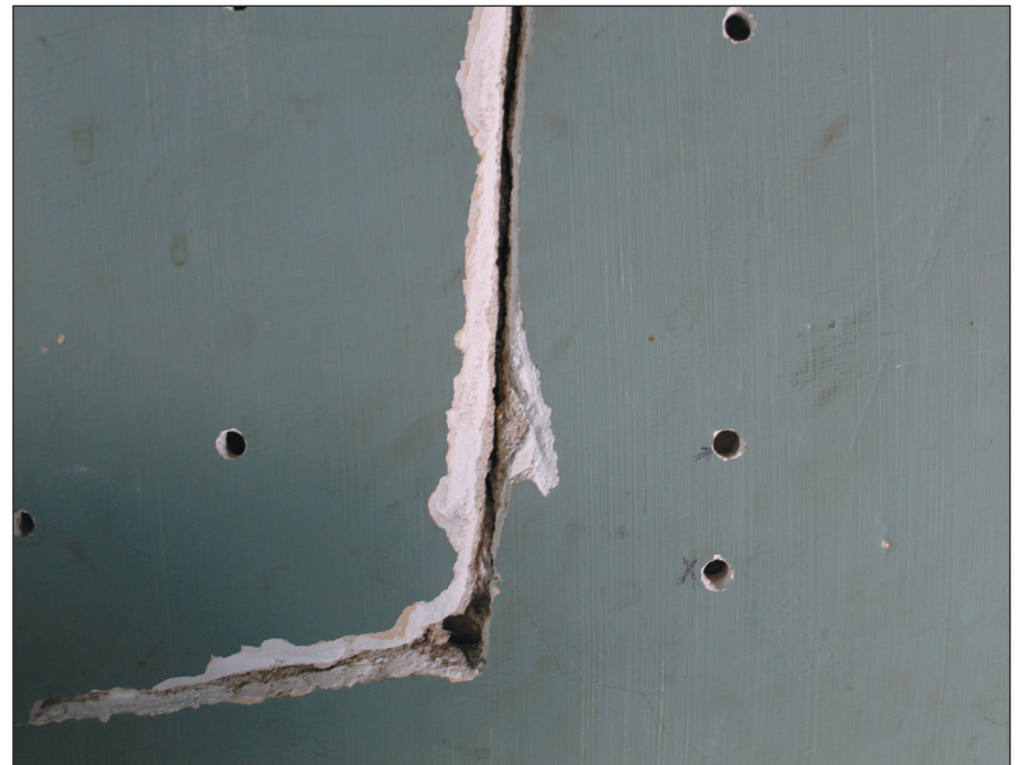
The crack has been vacuumed and holes drilled into the lath.
