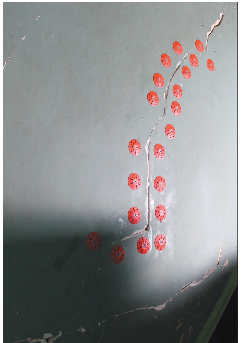
If you squint, it looks like a branch with flowers on it, right? The plaster is being stuck to the lath.
