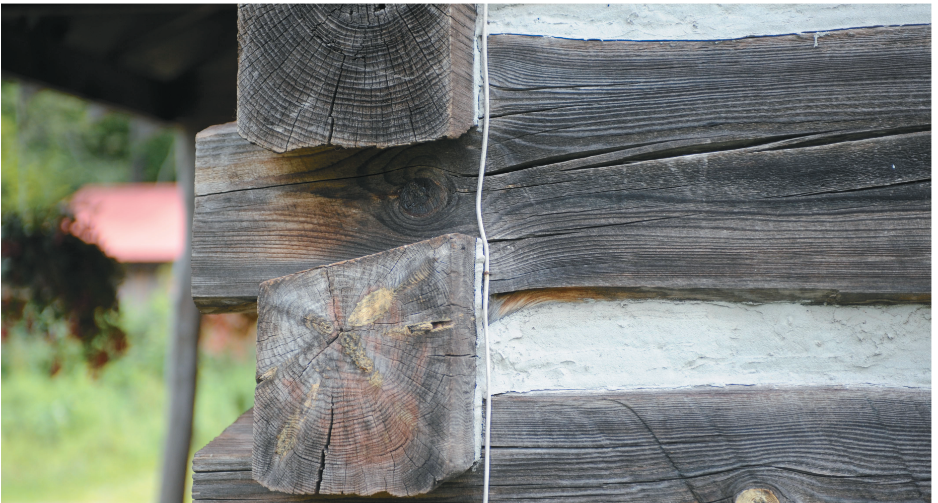
A detail of a corner of their Swedish-style log home, a design that interlocks the stacked logs, shears off water, and didn't use any nails except in the floors..
